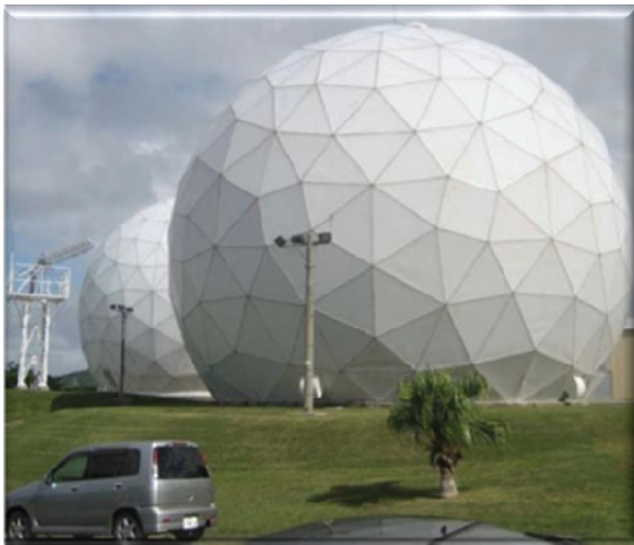
AFC's Two 68-ft diameter thin membrane wall DSF radomes for the Defense Satellite Communications System (DSCS), Okinawa, Japan.
